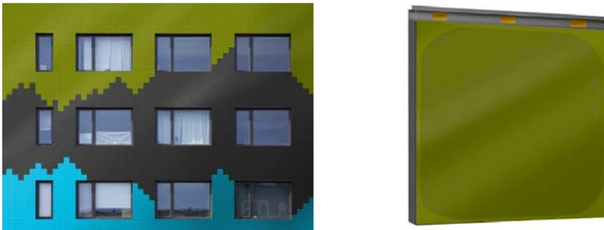
**Figure 1:** Facade with aesthetic solar modules and a single solar module (15x15cm)
