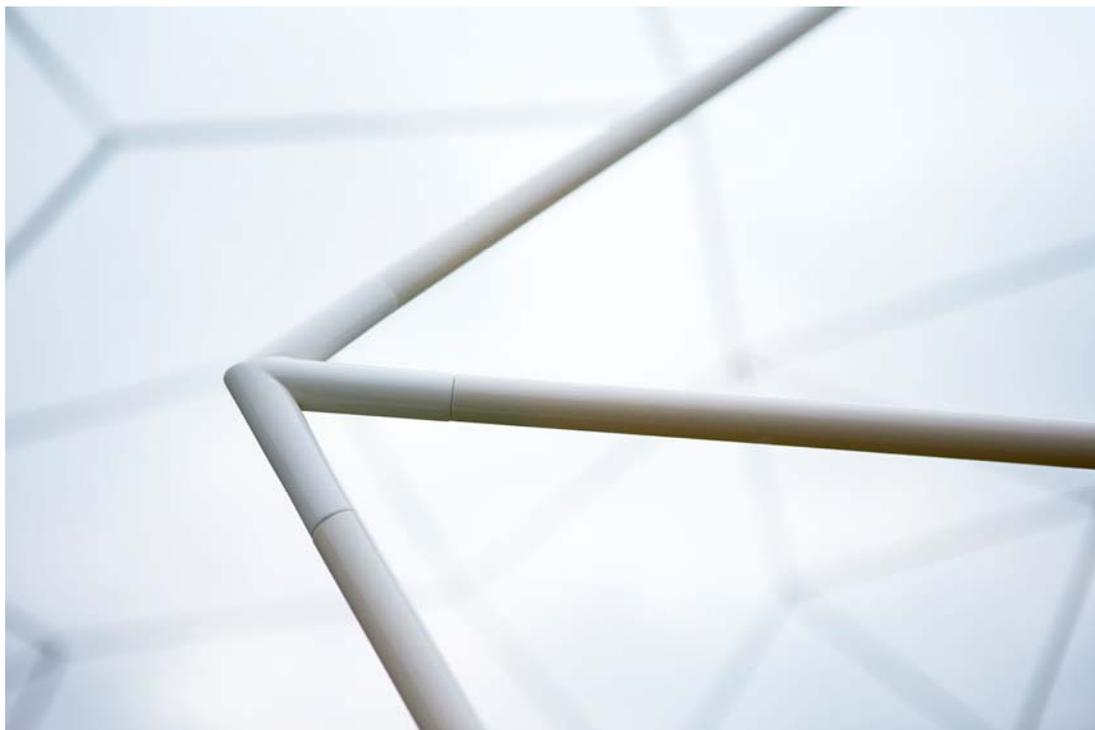
**Figure 6.** Photo of 3D-Printed Node Connection
