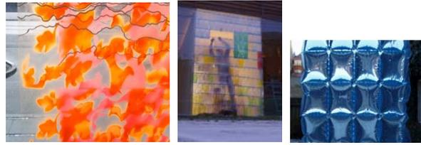
**Figure 5.** Constructions in EX 1, ice-cube bags and ornamentation imitating red colour pigment in PEC solar cell technology. Illustrates how solar cell technology can affect daylight in the façades and interiors. (Hansen 2013)
