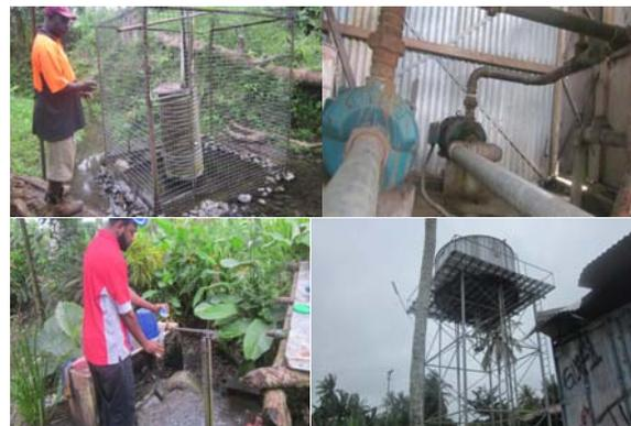
**Figure 11.** Pumping Station at Marthin Luther Seminary a) Suction Pump, b) 8000 Liters Reservoir
